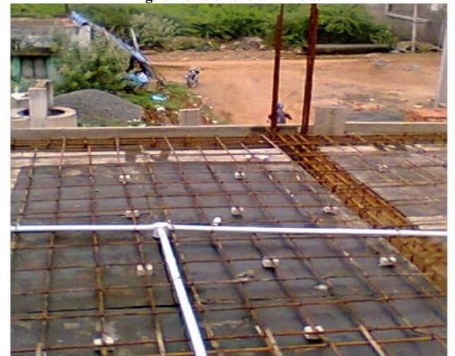
Fig.2. Reinforcement – One way slab
