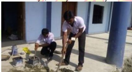
Fig.2.Mortar filling and Compaction
